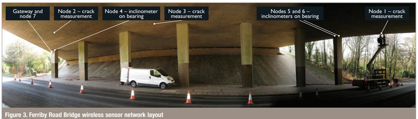
Figure 3. Ferriby Road Bridge wireless sensor network layout
