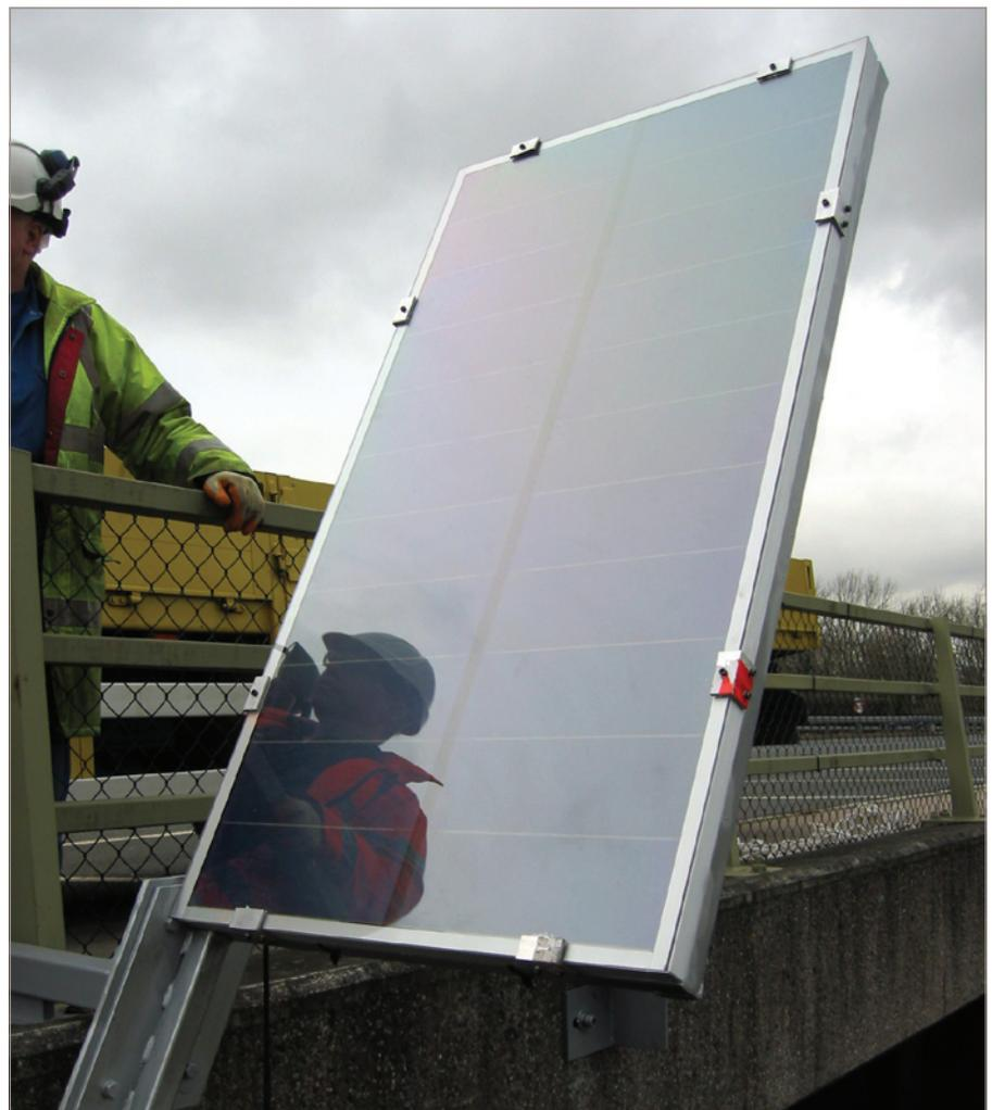
Figure 5. Solar panel attached to the side of the Ferriby Road Bridge to recharge the gateway's battery – this worked well in summer but only intermittently in winter
